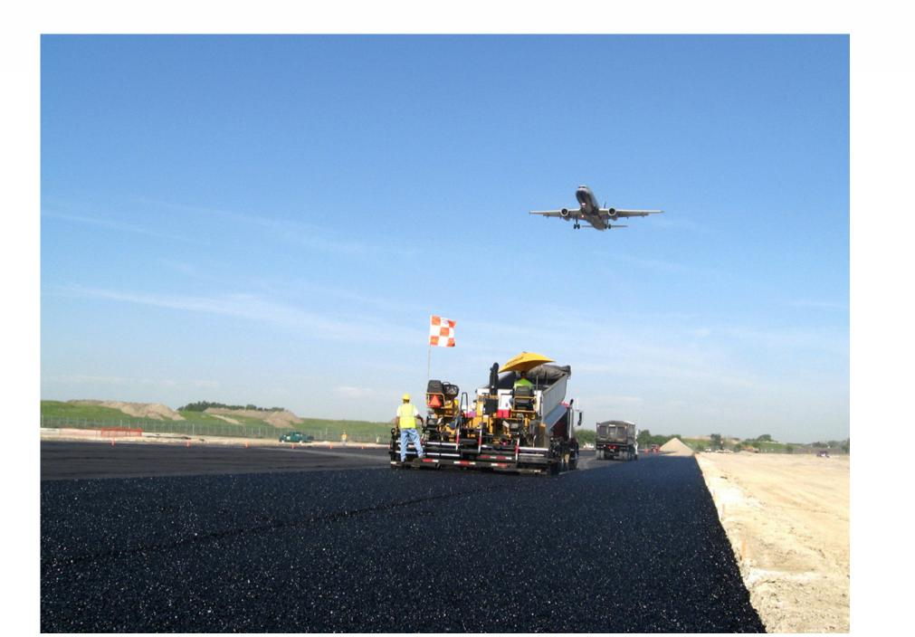
O'Hare International Airport is the first airport to recycle asphalt shingles. 8 million were kept out of the landfill and used in the construction of Runway 10R-28L.
